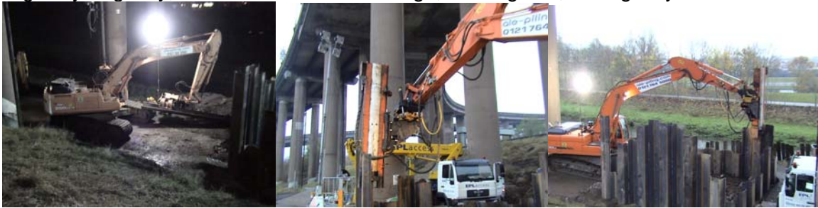
Highways Agency, M6-A38M Link Road Bridge, Birmingham, Emergency Cofferdam
