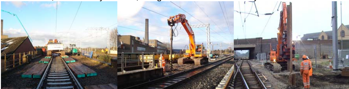
Network Rail, Trent Valley 4 Track, Bridge Abutments and Gantry Bases
