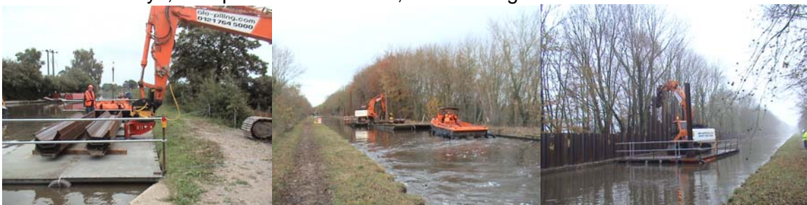
British Waterways, Shropshire Union Canal, Sheet Piling Embankment Afloat
