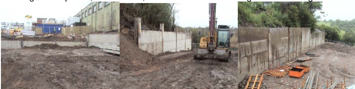
Housing Development, Manchester, Permanent Concrete King Post Retaining Wall
